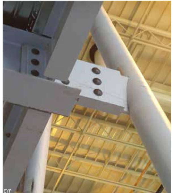
AESS connection of a floor beam to a truss diagonal.
